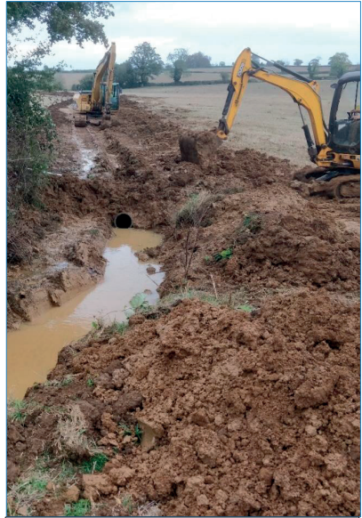
Field drain during construction
